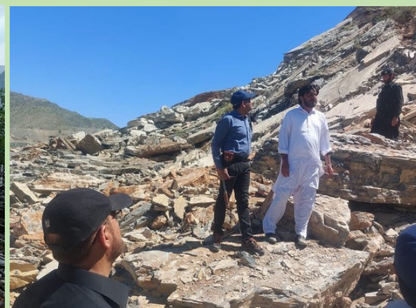
A GSP team visits and inspects the site of the devastating Torkham Landslide, which occurred on April 18, 2023, and claimed the lives of seven people.
