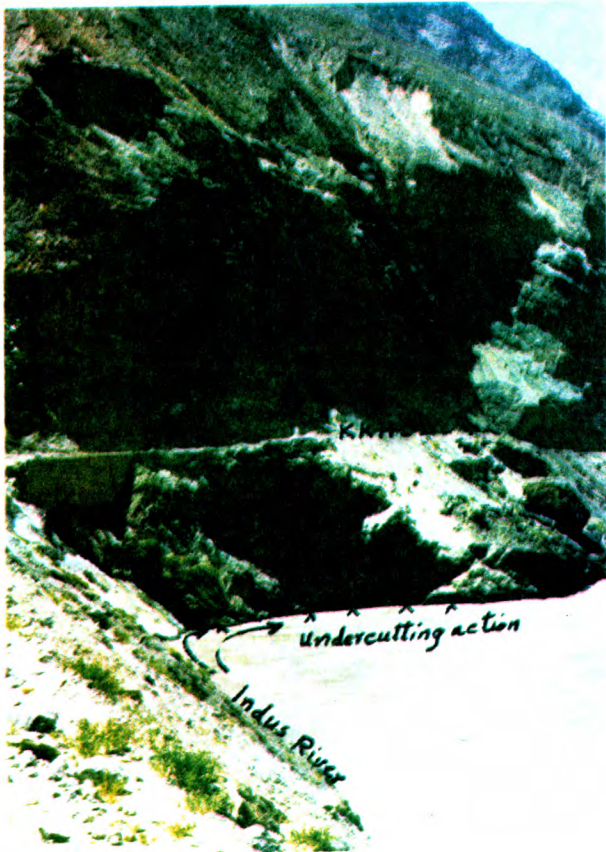
PLATE - 53 Road sinking problem in the zone of subsidence of the Tatta Pani area due to the presence of an active fault.
