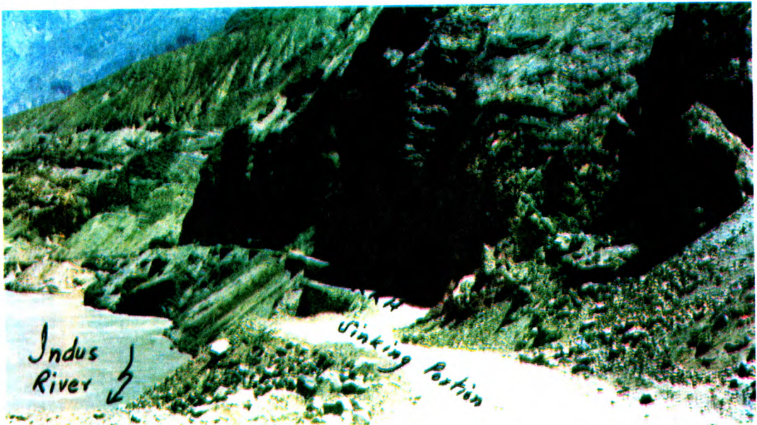
PLATE - 53 Road sinking problem in the zone of subsidence of the Tatta Pani area due to the presence of an active fault.
