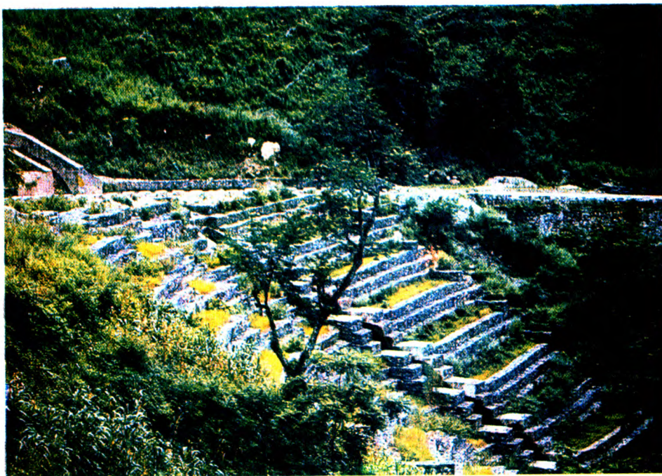
Plate - 63 Terracing of slope below road and grass painting. (Courtesy ICIMOD)
