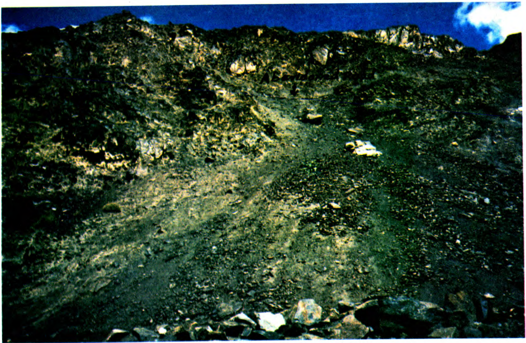
PLATE - 6 A view of GSP slide No. 3. Showing abandoned road in the centre of the slide.
