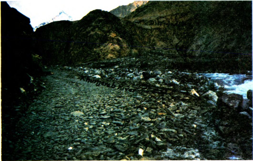
PLATE - 10 A view of Deh mudflow / avalanche site at the confluence of Khunjerab River with the source nullah at right corner.
