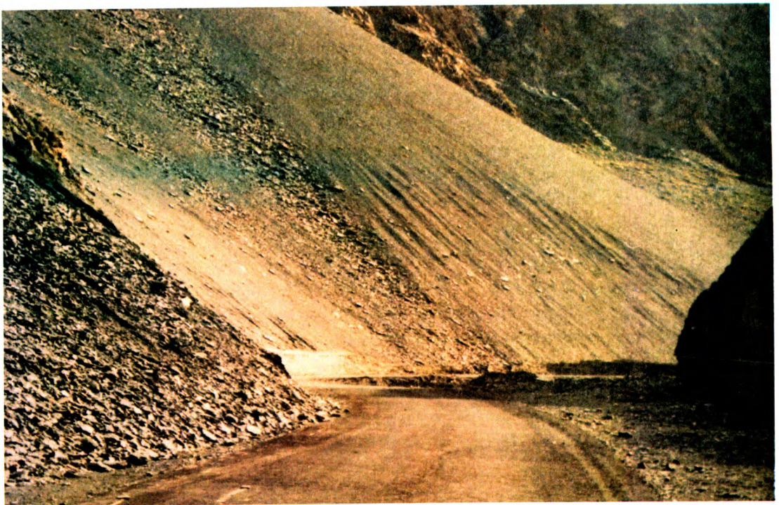
PLATE - 26 Overflow of scree from the breast wall.
