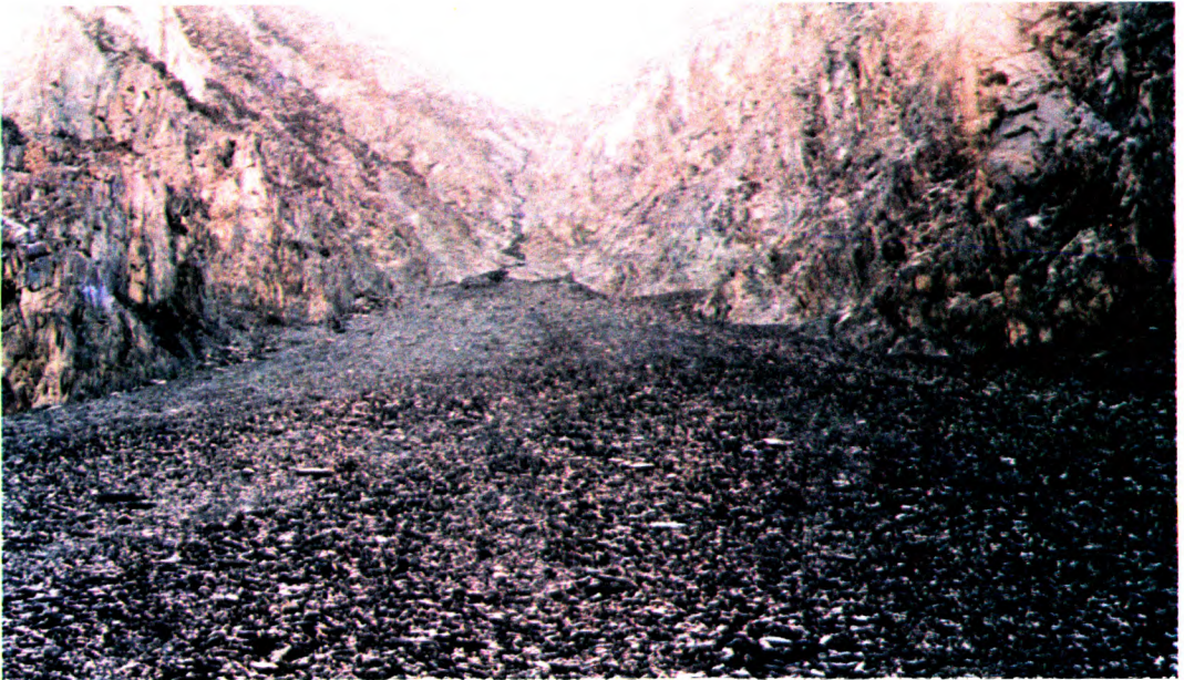
PLATE - 21 Debris slide are very common along the Karakoram Highway (KKH). Deeply weathered slate rocks and colluvium resulting from the disintegration of rocks in situ are lying at their critical angle of repose. Notice the angular fragments.
