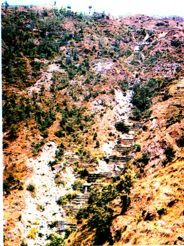
Plate - 65 A symbolic representation of a series of check dams or dykes constructed to reduce the impact of a rapid mudflow. (Courtesy ICIMOD)
