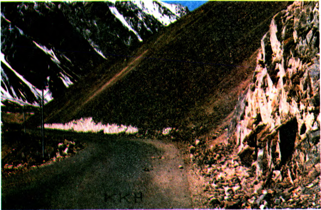
PLATE - 1 Scree slopes at their critical angle of repose causing hazards on road due to creep movement.
