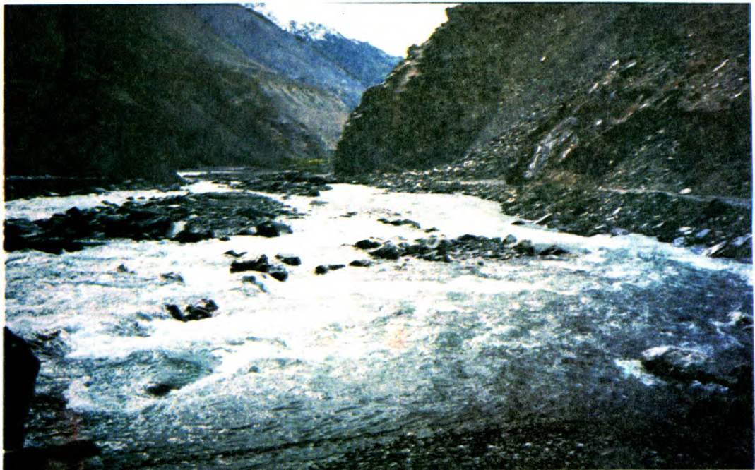
PLATE - 11 Deh avalanche looking down stream showing the damaged portion of the KKH on the right bank.
