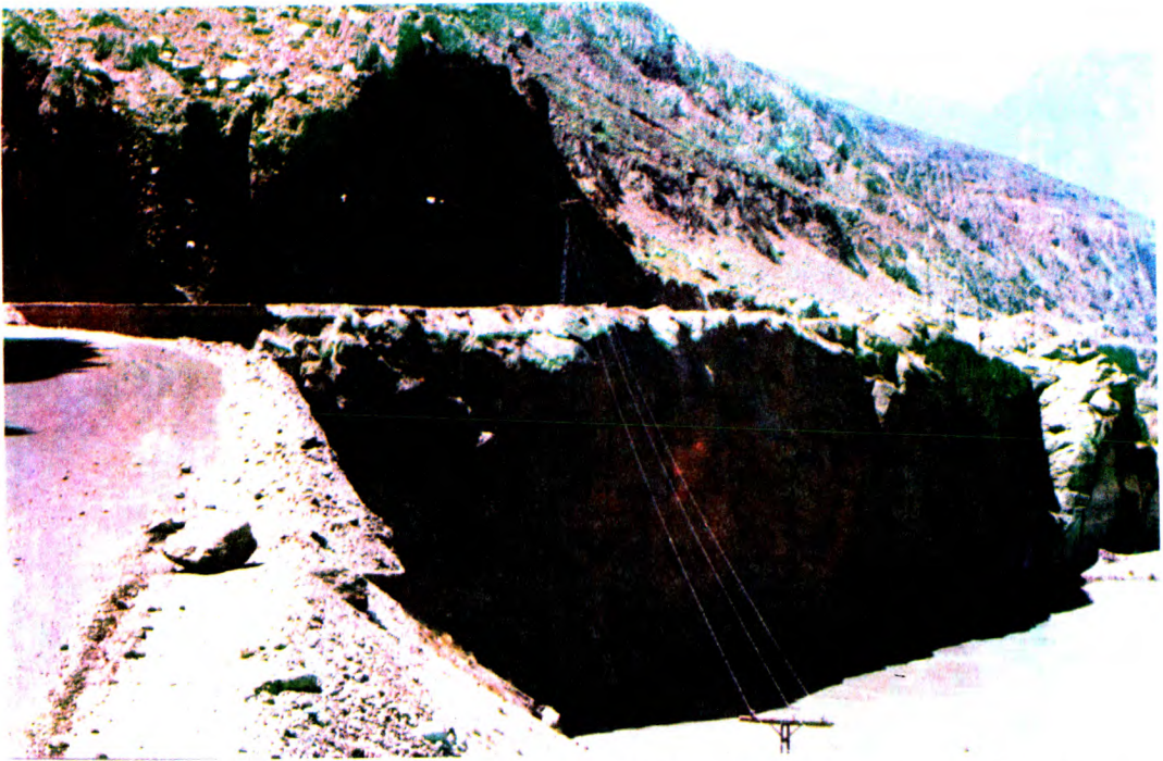
PLATE - 57 Vertically cliff face along the KKH at Gandlo as result of under-cutting action of the River. Bif boulders hanging precariously.
