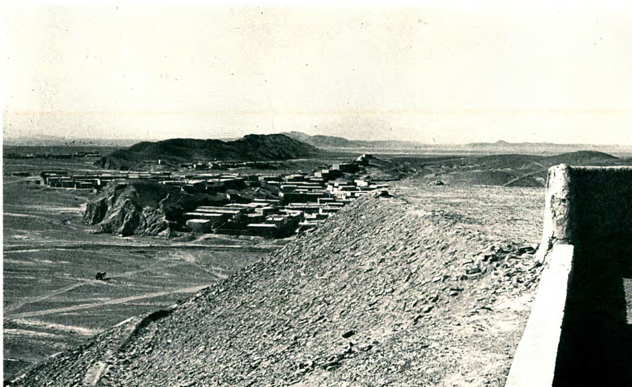
Figure 2. View looking south along the Chaman Fault from the top of the pressure ridge at Nushki. These ridges are formed of Quaternary sands and gravels squeezed up along the active fault zone. At the east edge of the ridge beside the small village of Faqir Kili these young gravels dip 70° east.
